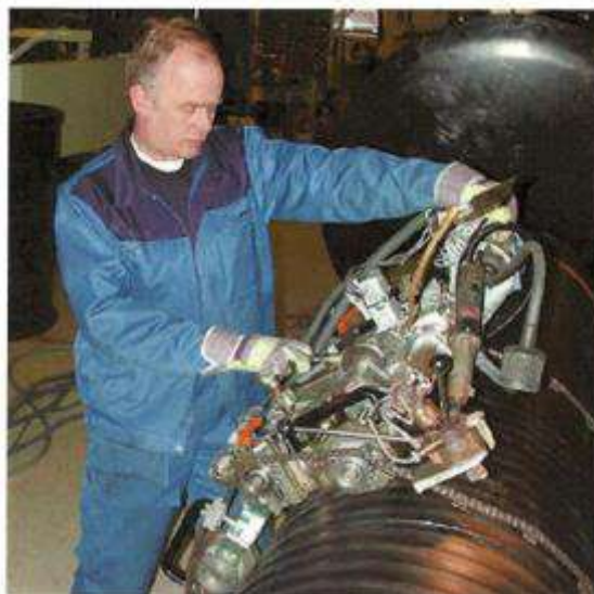
Figura 31 - Soldadura mediante máquina de soldar externa Figure 31 - Welding by external welding machine
