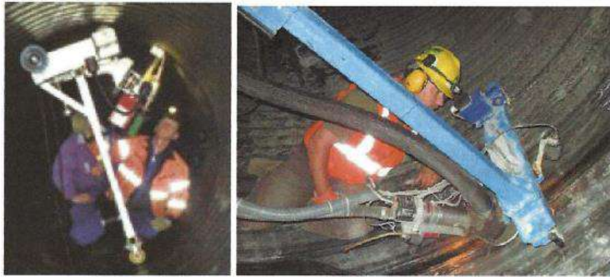
Figura 30 - Soldadura mediante máquina de soldar interna Figure 30 - Welding by internal welding machine
